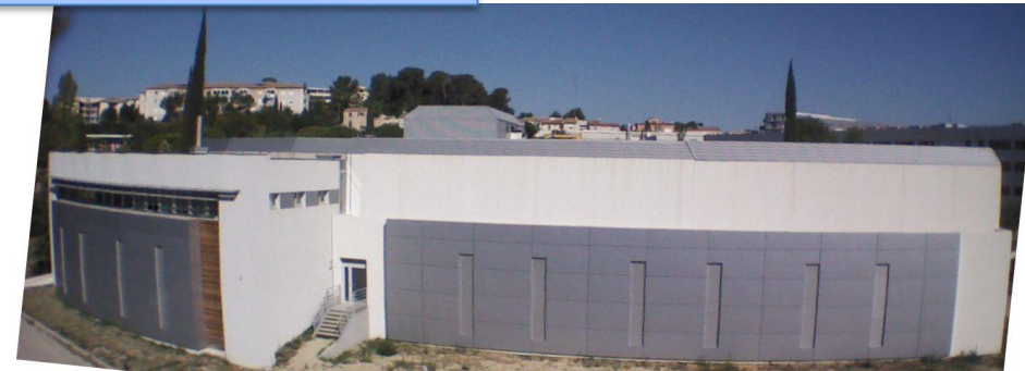
Dedicated machine room for Occigen: 600 m 2
